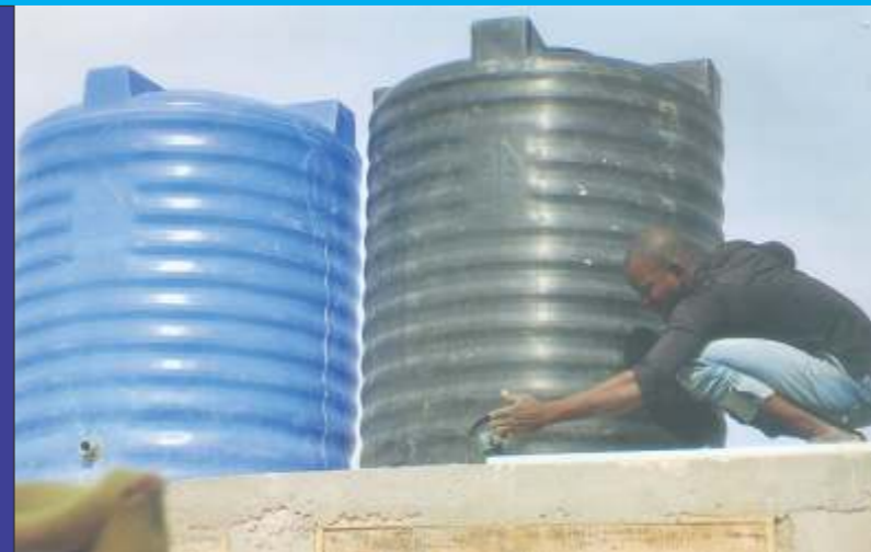
Constructed borehole and tanks supplied to the community of Allah gada, Ikara Local Government Kaduna State by ASD foundation, in the year 2018
