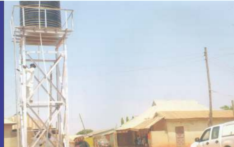
Constructed and donated borehole to Regasa Community (Zaria Road) in the year 2018 .by ASD Foundation
